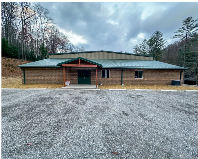
Construction on the Sunny Day Activity Center is almost complete!
