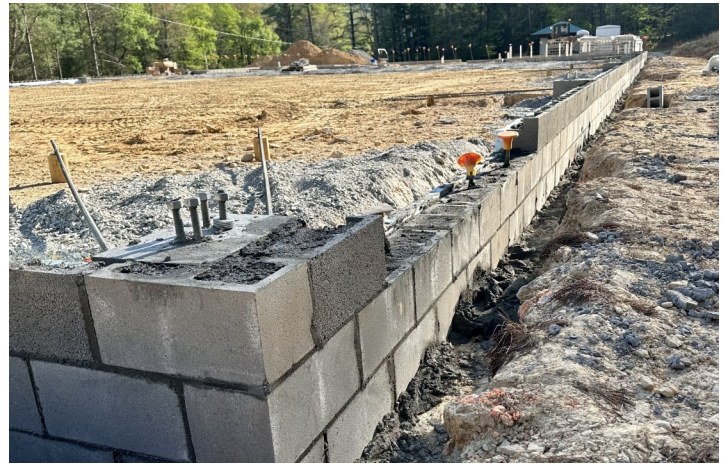
Installation of the masonry for the foundation stem walls.
